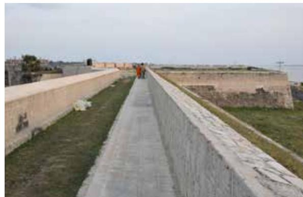
Fig. 53 Upper part of outer wall of the fort after restoration
